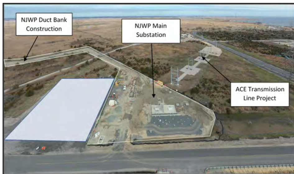
Figure 1. NJWP Parcel A construction progress (Photo Courtesy of AECOM-Tishman)
